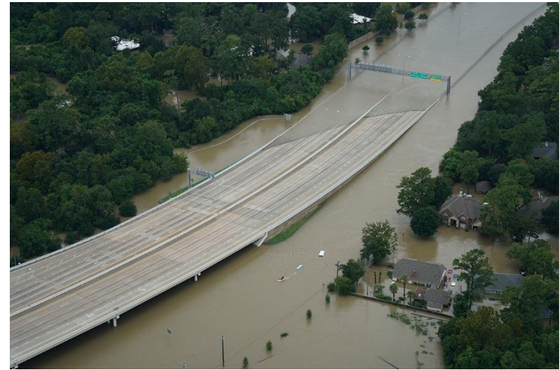
Flooding from Hurricane Harvey, Credit: TTI
